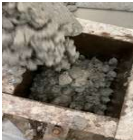
Figure 5: Concrete in mould
