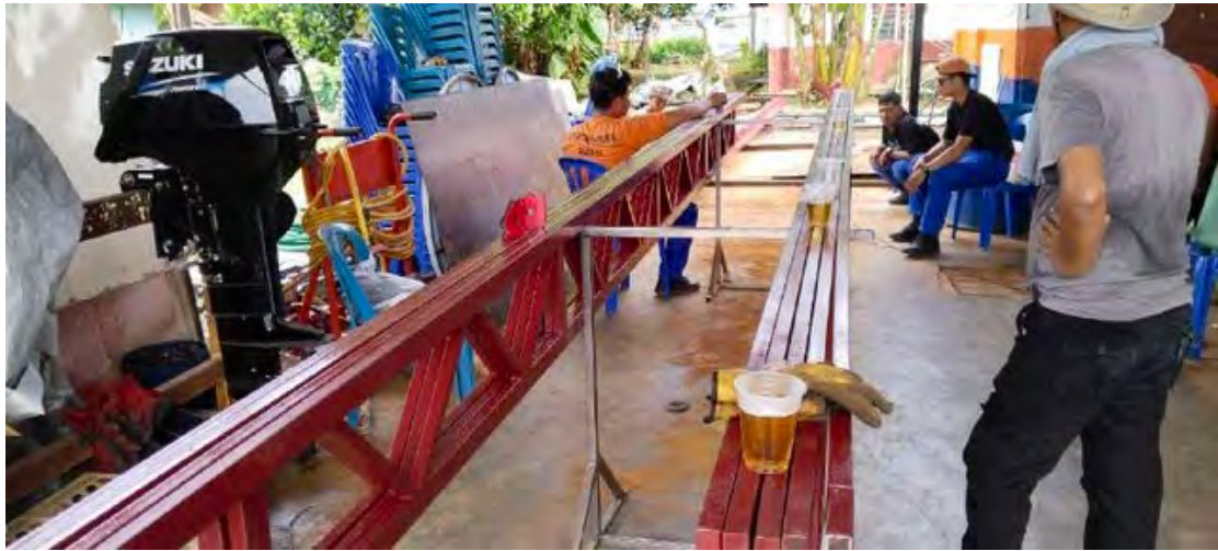
Rajah 19 Kursus Shielded Metal ARC Welding SMAW For Fillet Weld 3F.
