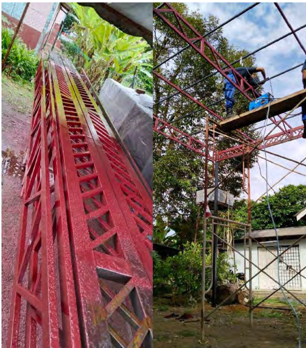
Rajah 21 Kursus Shielded Metal ARC Welding SMAW For Butt Weld 1G & 2G.
