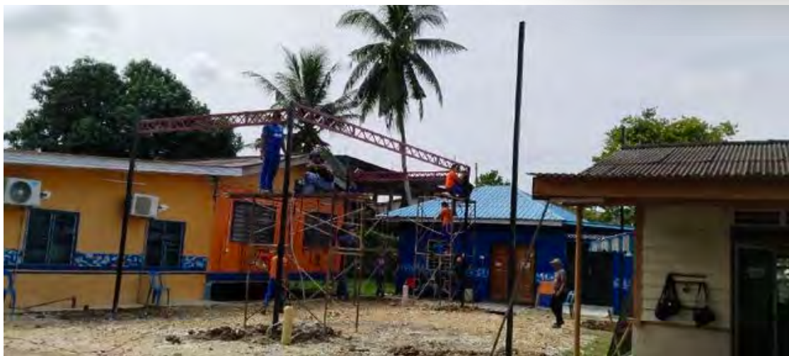
Rajah 17 Kursus Shielded Metal ARC Welding SMAW For Fillet Weld 1F.
